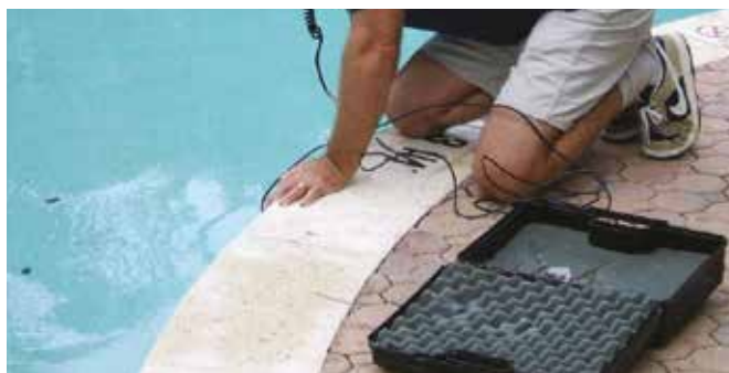
Leak detection, and Rectification
